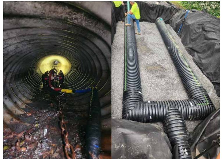
Phase 1 - Storm Sewer Cleaning and Televising
