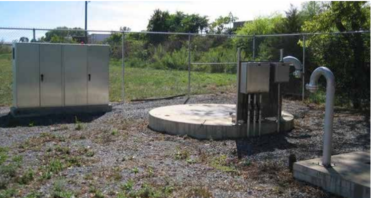
Typical Sewage Pump Station
